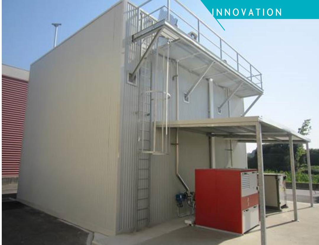
Exterior appearance of the building that houses the buried homogenization tank and the two ELAN® reactors of which the project consists.
